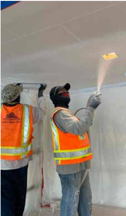
Adhering to COVID guidelines, two construction workers spraying plaster.
