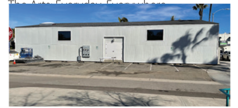
BEFORE: West Wall, 2787 State Street, Carlsbad, CA 92008
