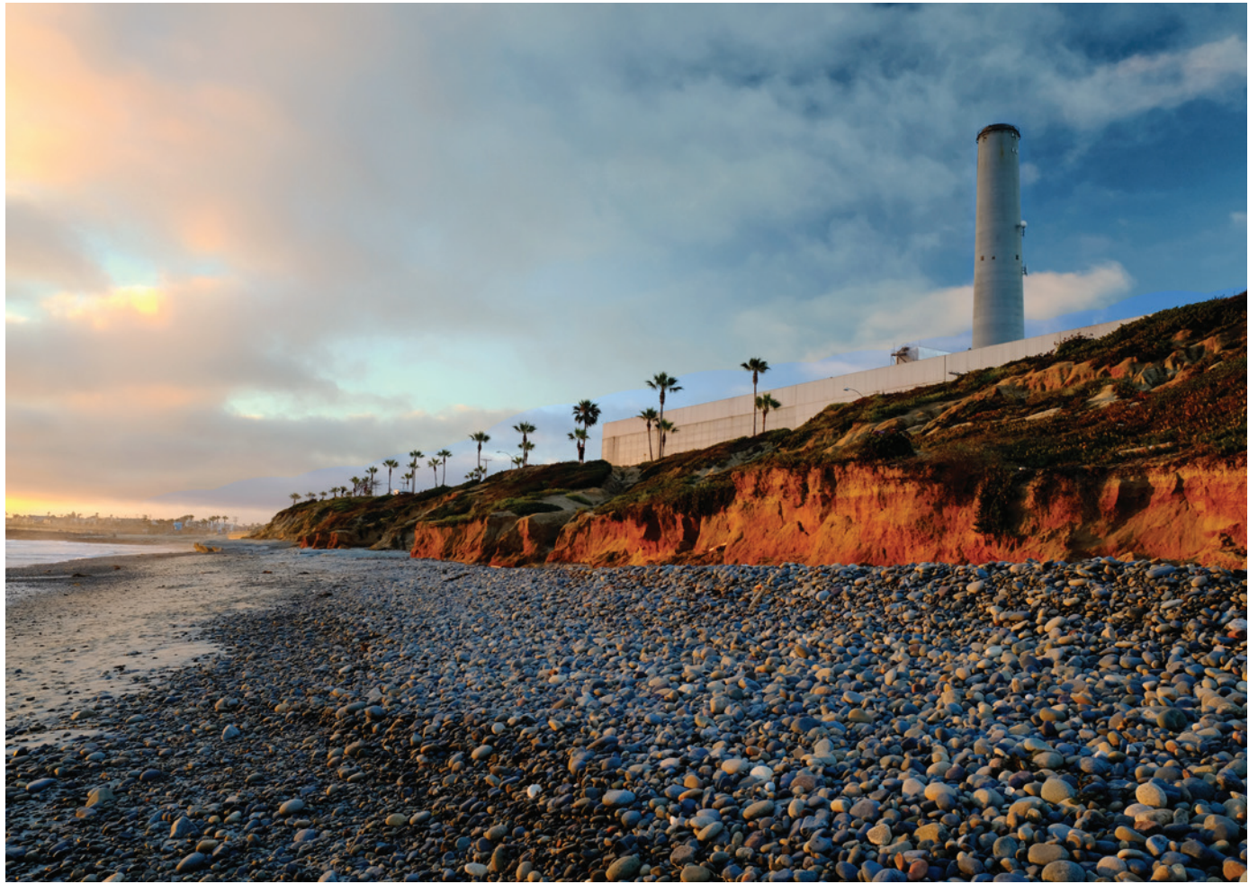
The Encina Power Plant (our long-standing smoke stack) was the flash point that pushed our community to incorporate.
