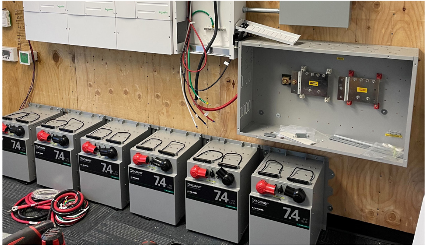
20kW Schneider Inverter System @ 208VAC with 38.4kWh Lithium (LFP) Battery Storage – installed in Thousand Oaks, CA
