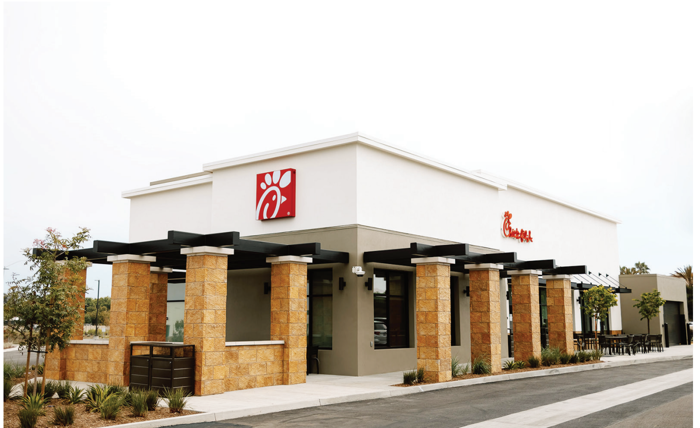
Located at 5848 Avenida Encinas, Chick-fil-A Carlsbad West will be open for dine-in, carry-out, catering pickup and delivery from 6:30 a.m. to 10 p.m., Monday through Saturday.
